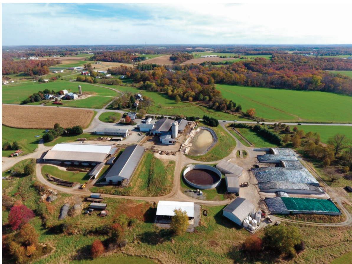
Chrome-View Farm is located near Nottingham in the southwestern corner of Chester County. Most of the over 700
